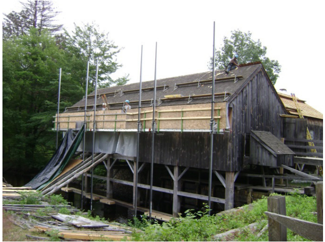
Our donors supported the Sawmill project, which included re-roofing.
